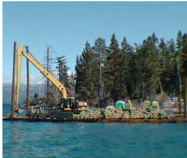
Surface operations during the deployment of benthic mats in Emerald Bay. Photo credit: B. Allen
