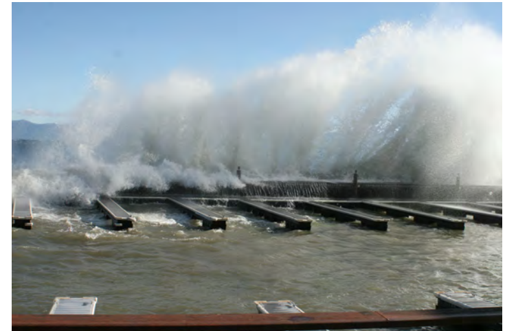
Waves breaking over Obexer's Marina with a strong easterly wind. Photo: D. Kramer
