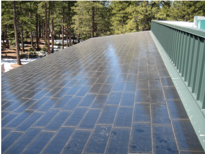
Photovoltaic Solar Panels (roof)
