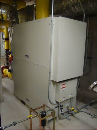
Gas-powered Microturbine
