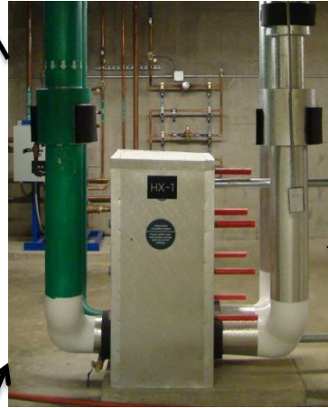
Heat Exchanger (HX-1; basement)
