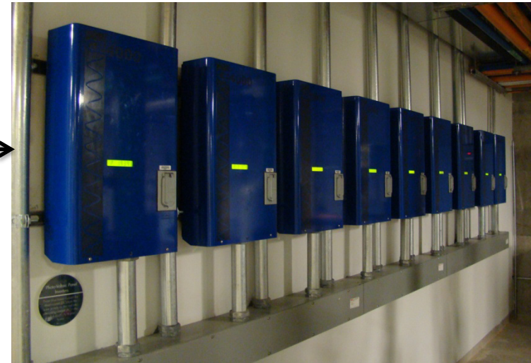
Photovoltaic Panel Inverters (basement)
