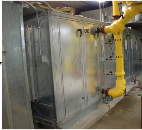
Filter and Humidifier (basement)
