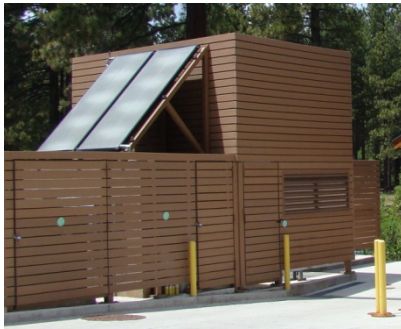
Evaporative Cooling Tower (Trex enclosure)
