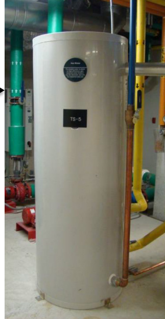
Hot Water Storage Tank
