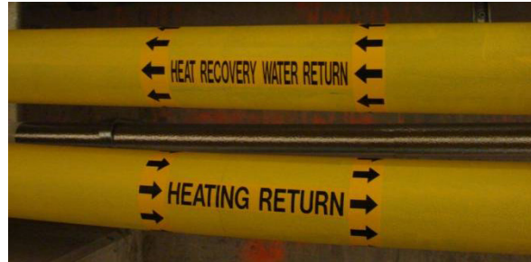
Heated Ethylene Glycol Pipes
