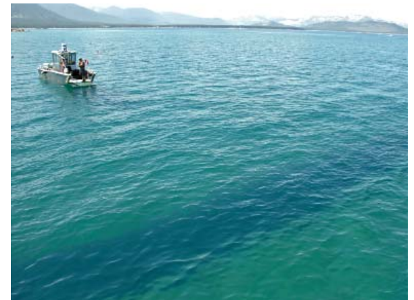
The first 100 foot long strip of rubber mat laid out on the lake bottom is visible in Marla Bay on July 9, 2010.
